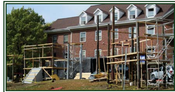
Lawn Display structures underway
